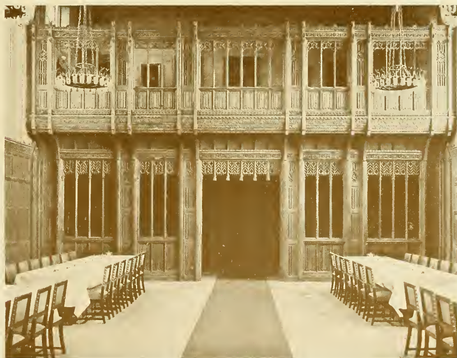
Detail of Great Hall, Princeton Graduate College Cram, Goodhue & Ferguson, Architects
